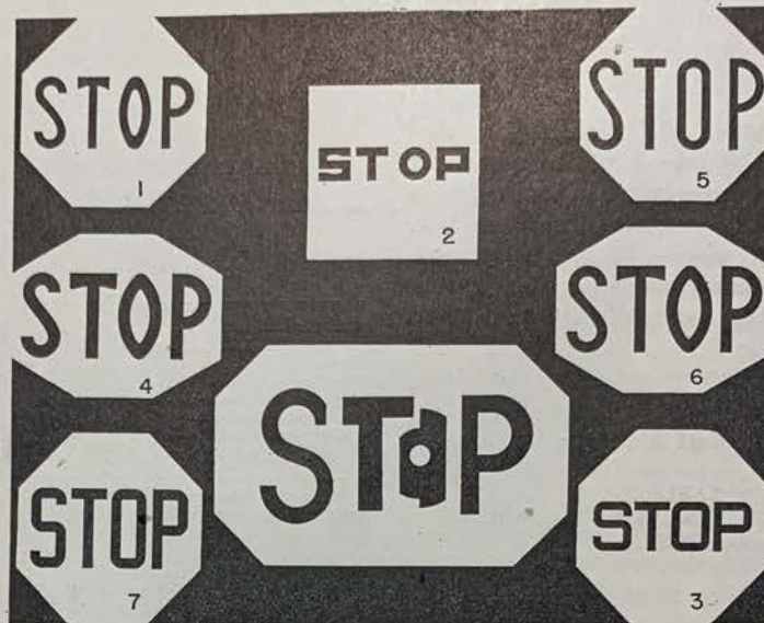
Figure 5. Types of Sign Studied—The sign at the lower left (No. 7) is a scaled reproduction from Neal of 30-in. stop signs used in Ohio. The sign at the lower right (No. 3) is a scaled reproduction of an older form of 24-in. stop sign used in Iowa. These are typical of signs being subjected to further analysis in various forms of reflectorization.
